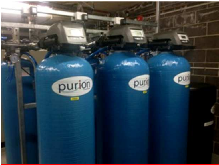
(A) 2 carbon filters, 1 softener tank and a brine tank in series.
