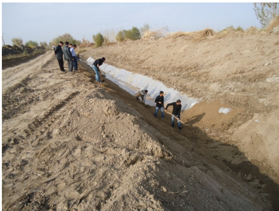
Figure 4. Covering of plastic with compacted soil
