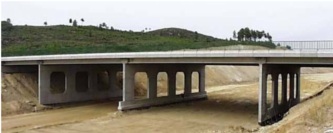
Figure 4. Overpass on A23 performed with prefabrication (Juntas, 2013)
