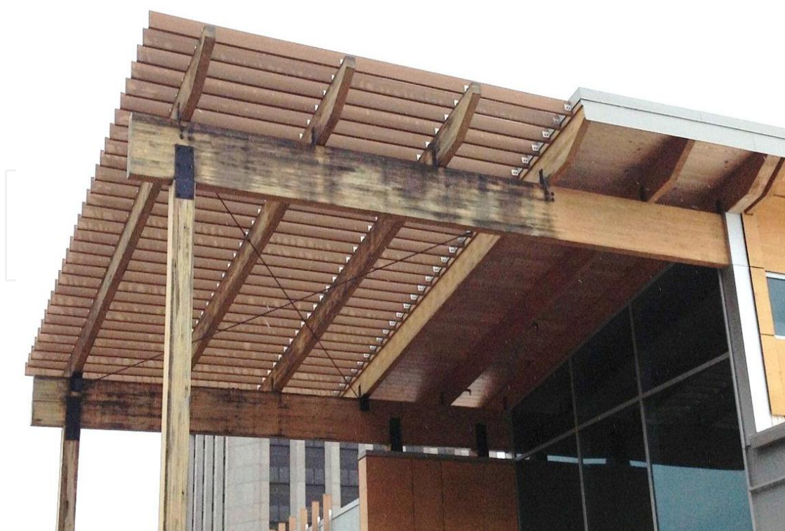
Figure 10. Illustration of the importance of roof overhangs for protecting wood from biodeterioration and corrosion. The right side of the beam is protected by the large roof overhang, whereas the left side is exposed to rain. SCALE: The beam supporting the trellis is 0.66 m deep.
