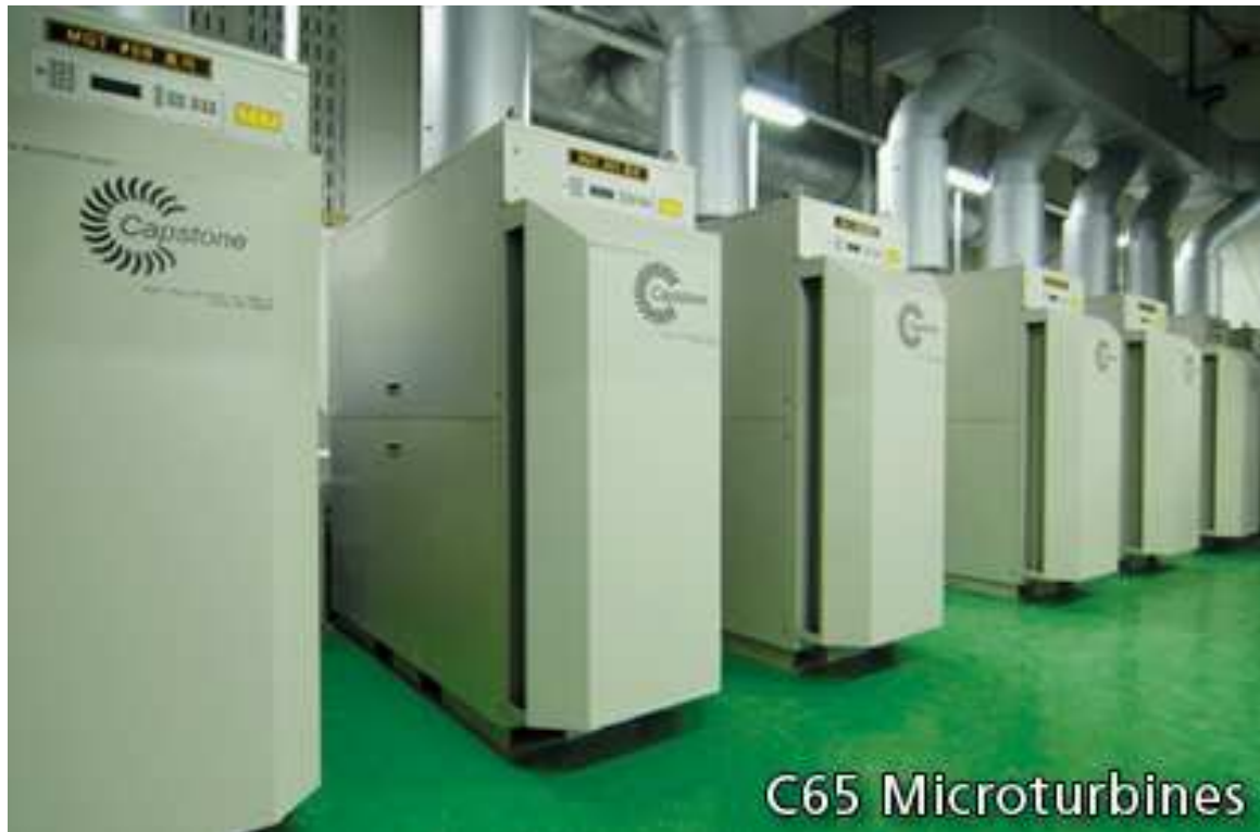
Figure 2. Capstone microturbine, model C65 (Capstone, 2012).
