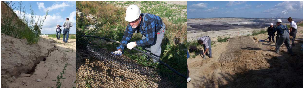
Figure 13. Installation of a geogrid containing PMMA POF at a creeping slope in a brown coal pit near Belchatow, Poland.
