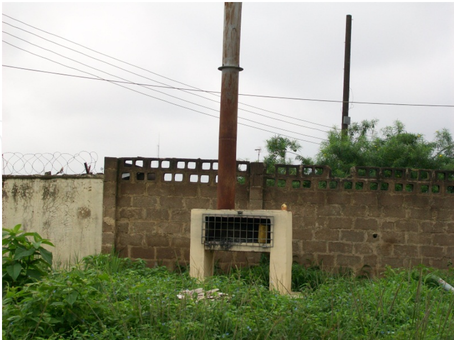
Figure 1. Locally developed incinerator using concrete
