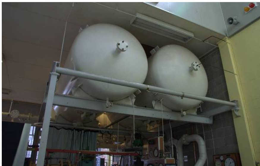
Figure 5. Air Storage Vessels
