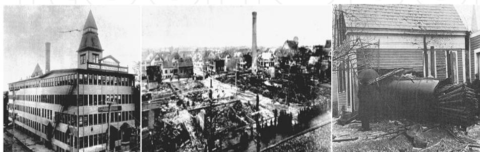
**Figure 1.** View of the R. B. Grover & Company Shoe Factory before (left) and after (middle and right) the boiler explosion on March 20, 1905, that killed 58 persons and injured 117, (USGenWeb, 2011, Ellenberger et al., 2004).
