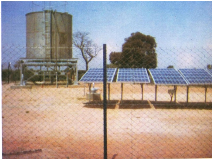
Figure 6. Photovoltaic water pumping station with a volumetric pump at Niger.
