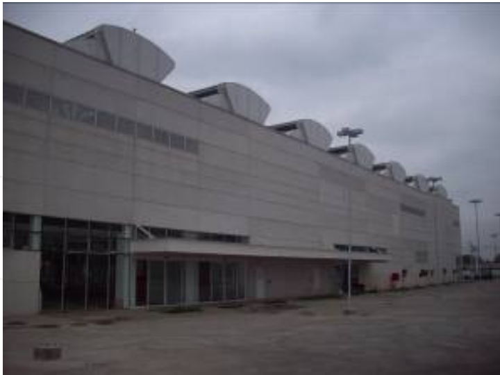
Figure 20. The Operational Support Building, one of the factory type buildings featuring triple floor to ceiling heights and shed structures in the roof for daylight and stack ventilation.
