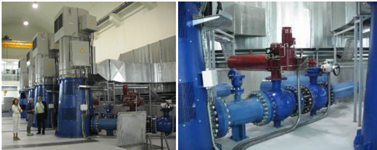
Figure 3. Socorridos pumping station: centrifugal pumps and control valves
