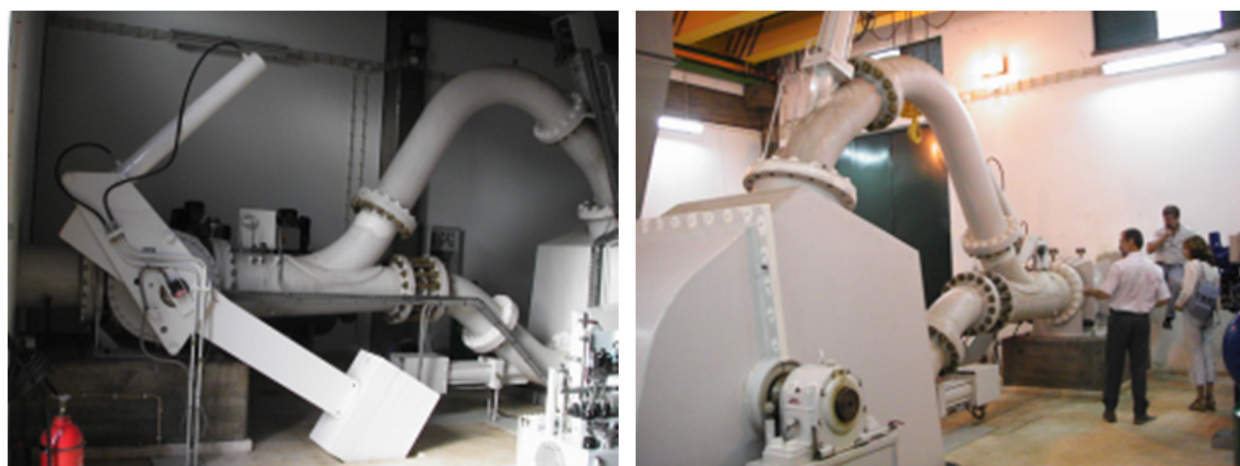
Figure 6. St. Quitéria hydropower station: inside view of Pelton turbine
