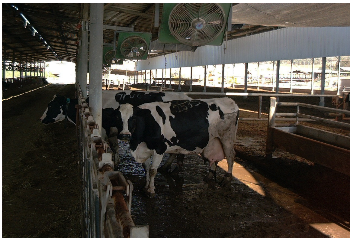
Figure 5. A cooling system based on spray and fans placed over the head-locks, next to the feedbunk.
