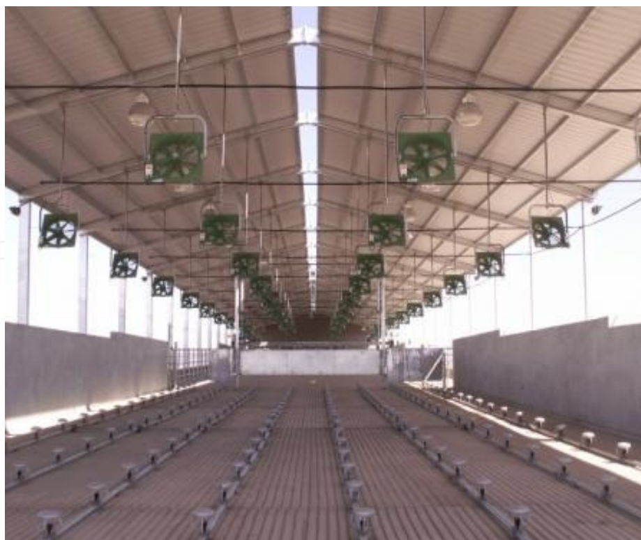
Figure 6. A cooling system based on spray and fans installed in the roof of the holding pen, prior to the milking parlor.
