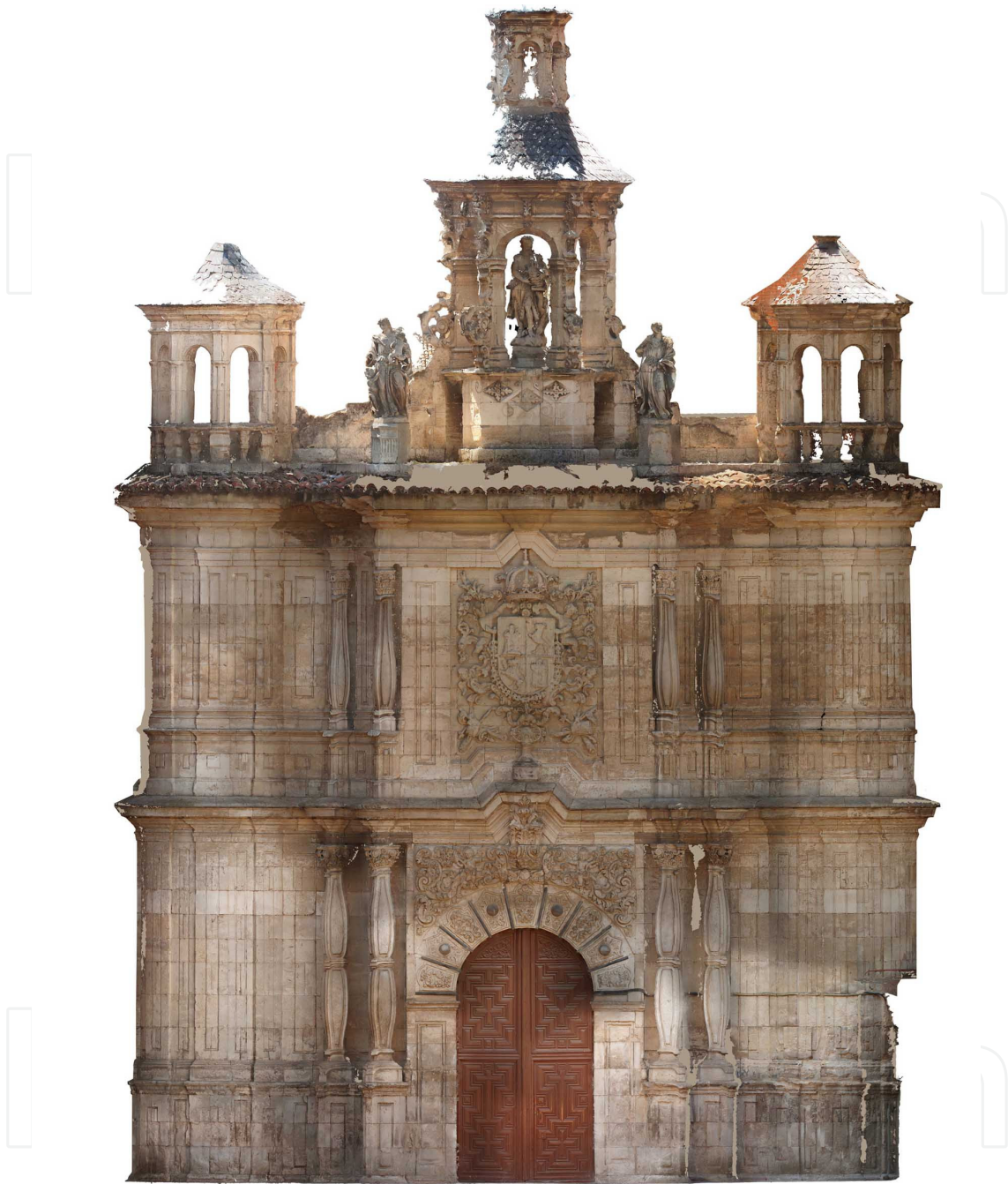
Figure 7. Texture and colour data of the façade of San Juan de Letran; example of compensated distortions of a photograph (Task Group's Partner: DAVAP Research Team , University of Valladolid, Spain).
