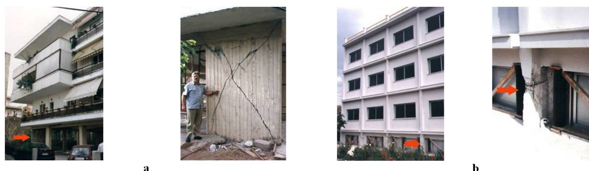
Figure 3. a Typical damage of shear walls at the “soft story” during The Kozani 1995 Earthquake in Greece. b. Typical damage of “short” columns during The Kozani 1995 Earthquake in Greece.
