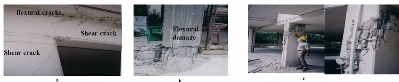
Figure 2. a Typical damage of beam at the joint with the nearby column (6 th story building, Aharnes, Athens earthquake 1995), [2]. b Typical damage of the toe of a column at ground floor (two-story building, Nea Kifisia,, Athens earthquake 1995), [2]. c Typical shear damage at the columns of a “soft story” (4-story Metamorfofi building, Athens earthquake 1995), [2].
