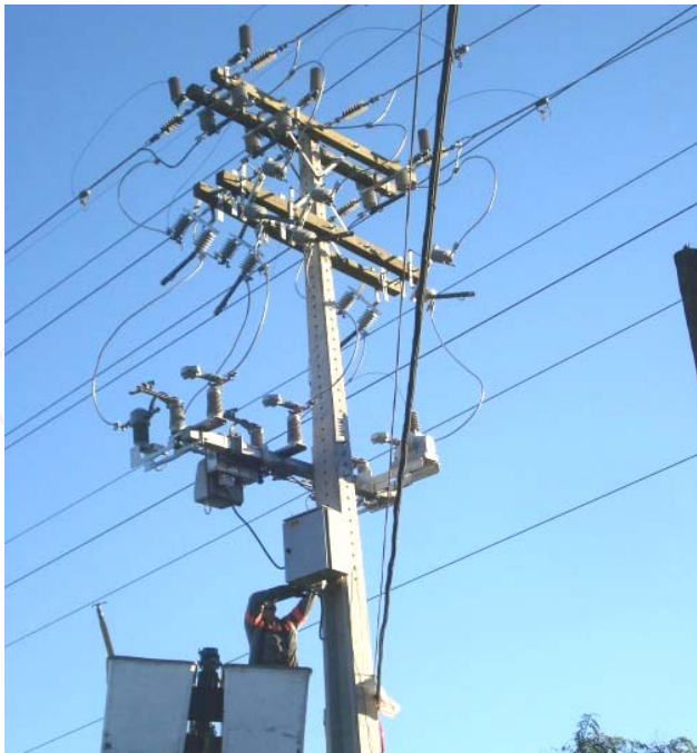
Fig. 8. Installation of a remote controlled switch.
