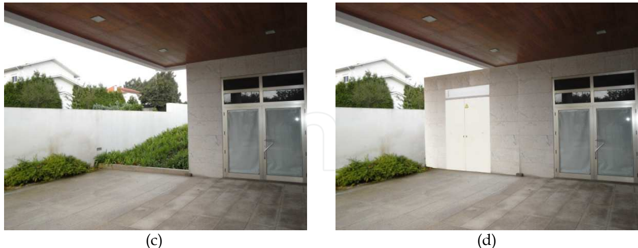
Fig. 12. Landscape integration of transformer stations in relation to structures (a) transformer station built-in a wall; (b) transformer station attached to an existing construction; (c) and (d) transformer station built by extending an existing building.
