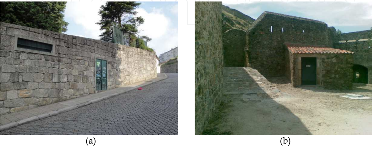
Fig. 11. Proposed integration of a substation in northern Portugal through terracing and planting schemes according to the character of the prevailing landscape
