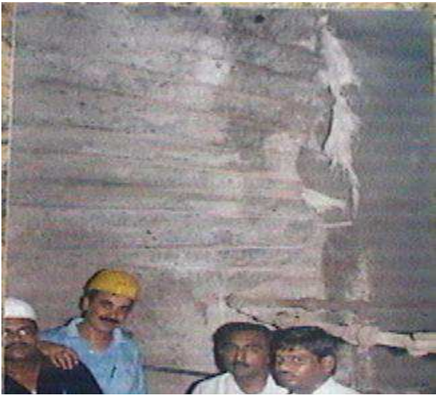
Fig. 5(b). Pier nose wall after pre-split blasting
