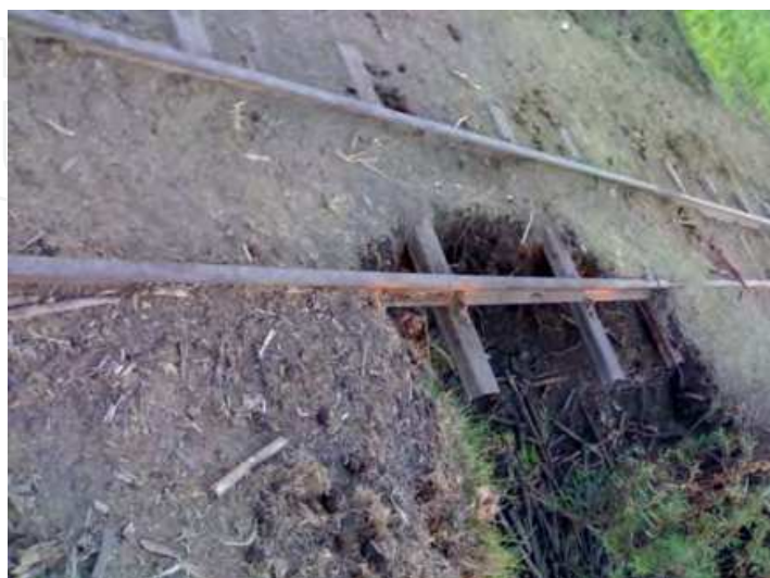
Fig. 17. Soil Erosion under the railroad.
