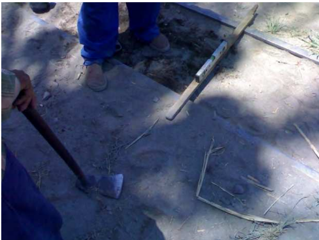
Fig. 22. Balancing the level of the rail track
