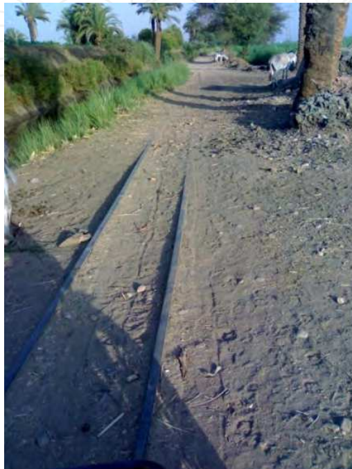
Fig. 18. The narrow railroad constructed on the middle of an infield road with parts covered with dirt
