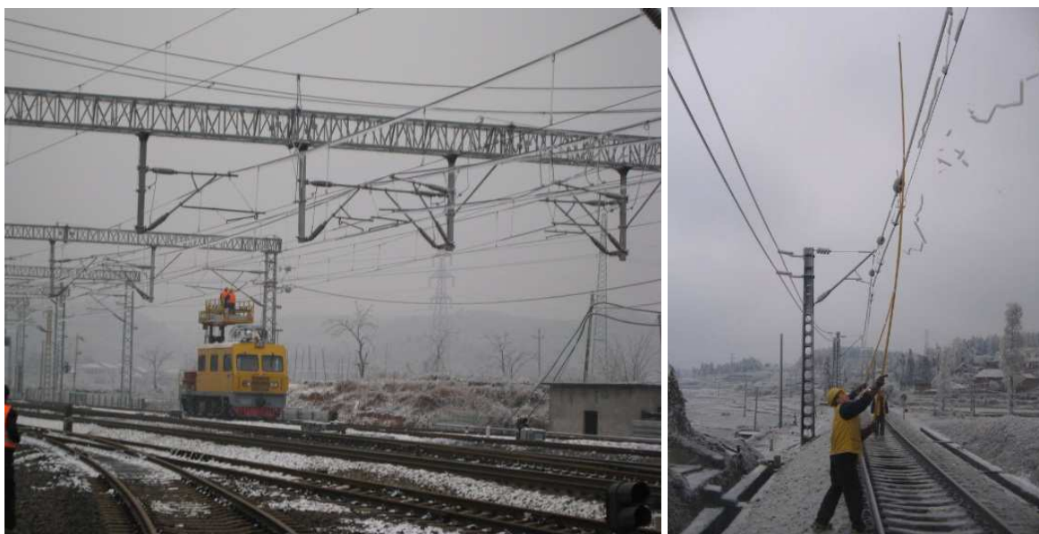
Fig. 1-1. Manual de-icing on overhead contact wires
