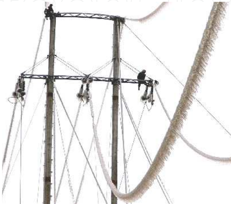
Fig. 2-1. Icing of high-voltage line
