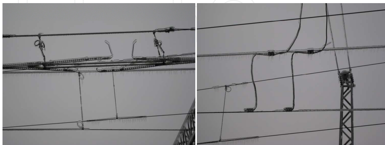
Fig. 1-2. Icing of overhead contact wire
