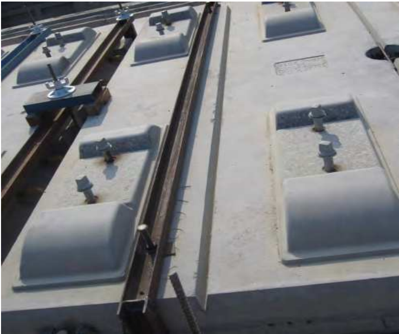
Fig. 33. Tight the slab track
