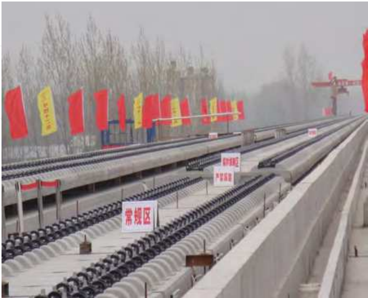
Fig. 31. Preparation before grouting
