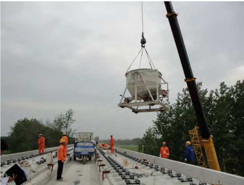
(b)Transportation of CA mortar
