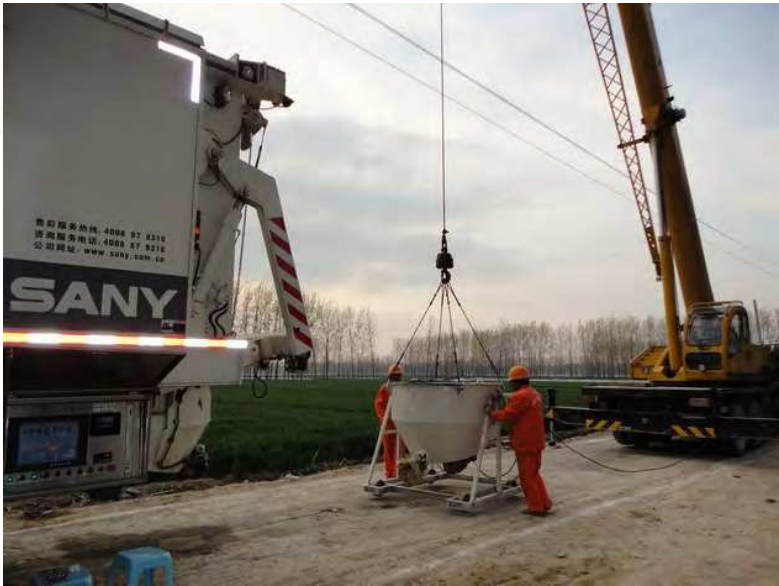
(a)Transportation of CA mortar
