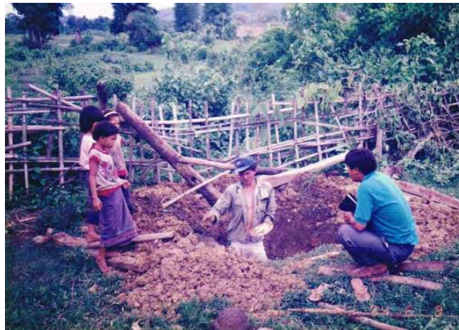
Picture 3. Making of pit for toilet
