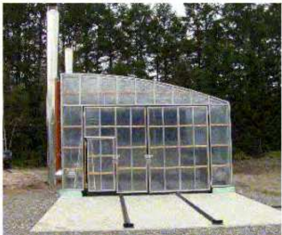
Photo 2. Front View of A Fully Passive-type Soalr Lumber Drying House; (East-West model)
