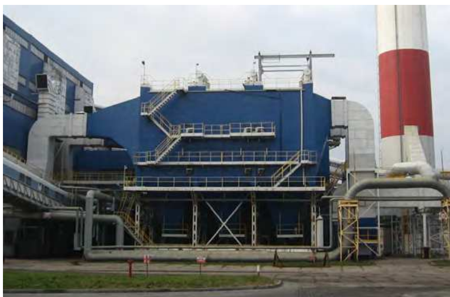
Fig. 1. Electrostatic precipitator in Thermal-Power Station.
