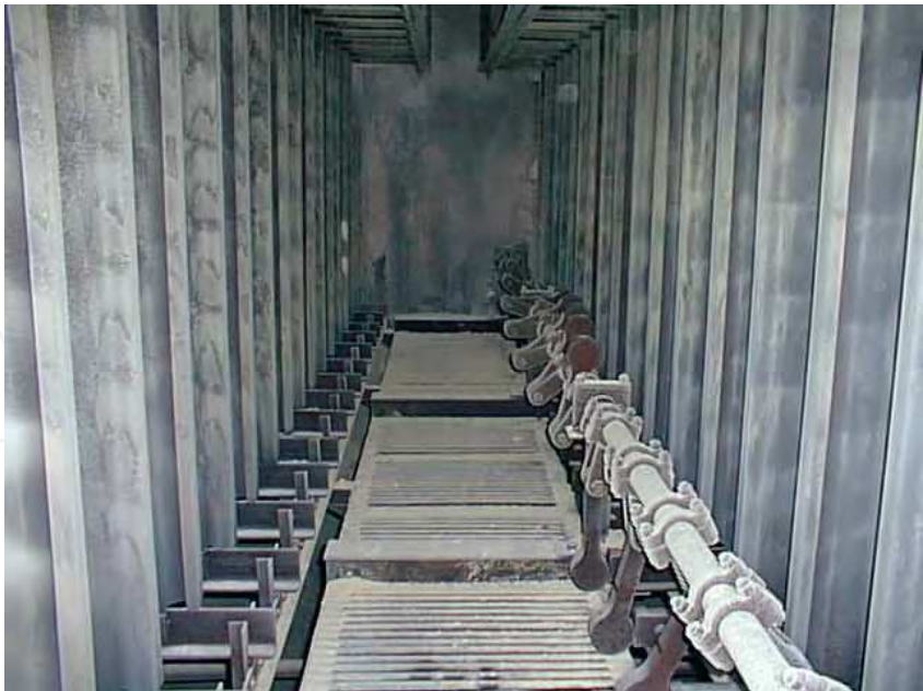
Fig. 2. Inner part of the ESP.
