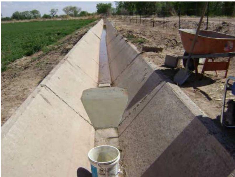
Fig. 5. Completed Broad Crested Weir for Field 3
