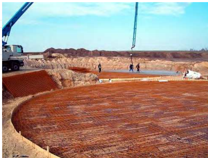
Fig. 8. Structuring the grid irons for a commercial biogas plant (MT-ENERGIE GmbH & Co. KG)
