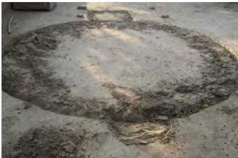
Fig. 5. Marking of dimensions for a biodigester
