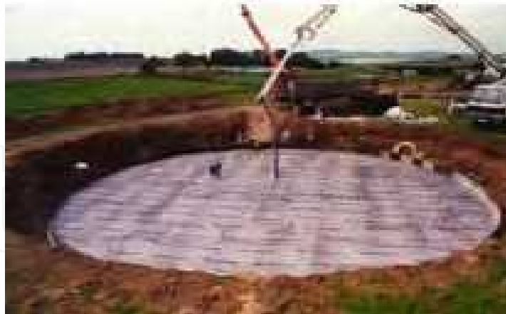
Fig. 9. Pouring the concrete mixture for a commercial biogas plant (BIOGAS NORD GmbH)
