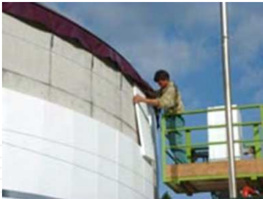
Fig. 17. Installing the insulation (BIOGAS NORD GmbH)
