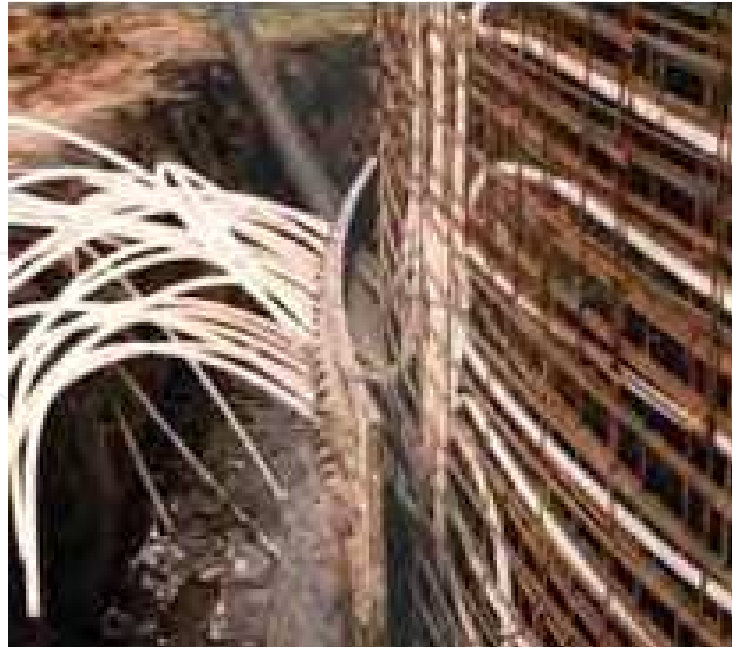
Fig. 13. Integrating the heating tubes (BIOGAS NORD GmbH)
