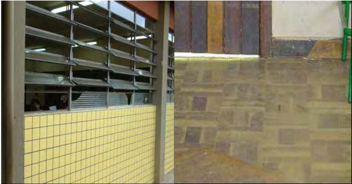
Fig. 18. Classroom com broken window panes and spaces between the door and the floor
