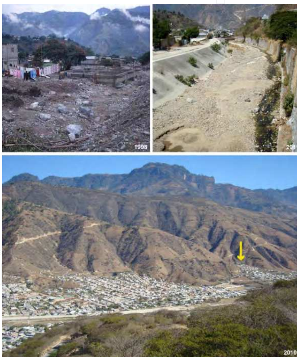
Fig. 14. A mostly dry channel of a tributary creek passing through Motozintla (upper left after the disaster in Sept. 1998, upper right in Feb. 2011 after channelling) and overview on those suburbs of the town which were installed mainly after the 1998 event; the yellow arrow marks a recently established quarter highly endangered by flash floods
