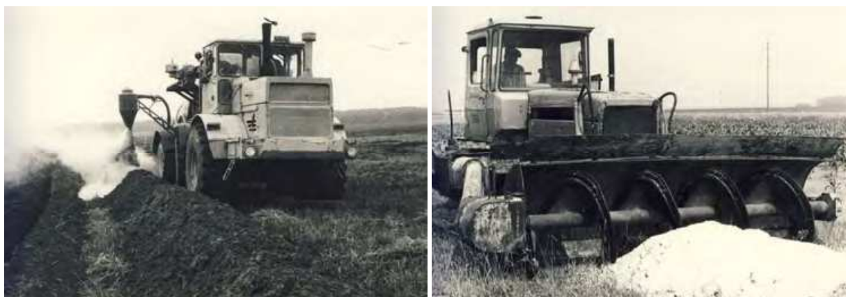
Fig. 3. Installation of lime filter drainage in Kalnūjai site
