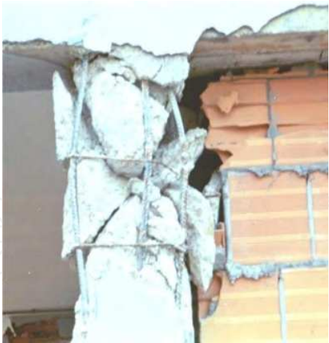
Fig. 9. Shear failure of column (Italia 2002)
