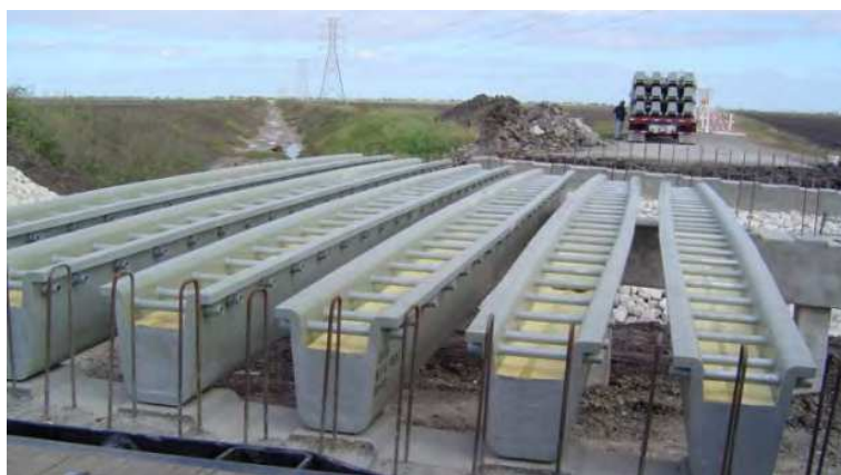
Fig. 16. Hybrid FRP/Reinforced Concrete Bridge Girders Evaluated with Acoustic Emission (after Ramirez et al., 2009)
