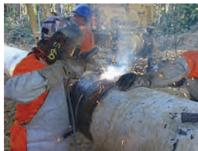
Fig. 30. Pipeline manual welding procedure.
