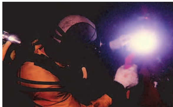
Fig. 2. Underwater welding with SMAW.
