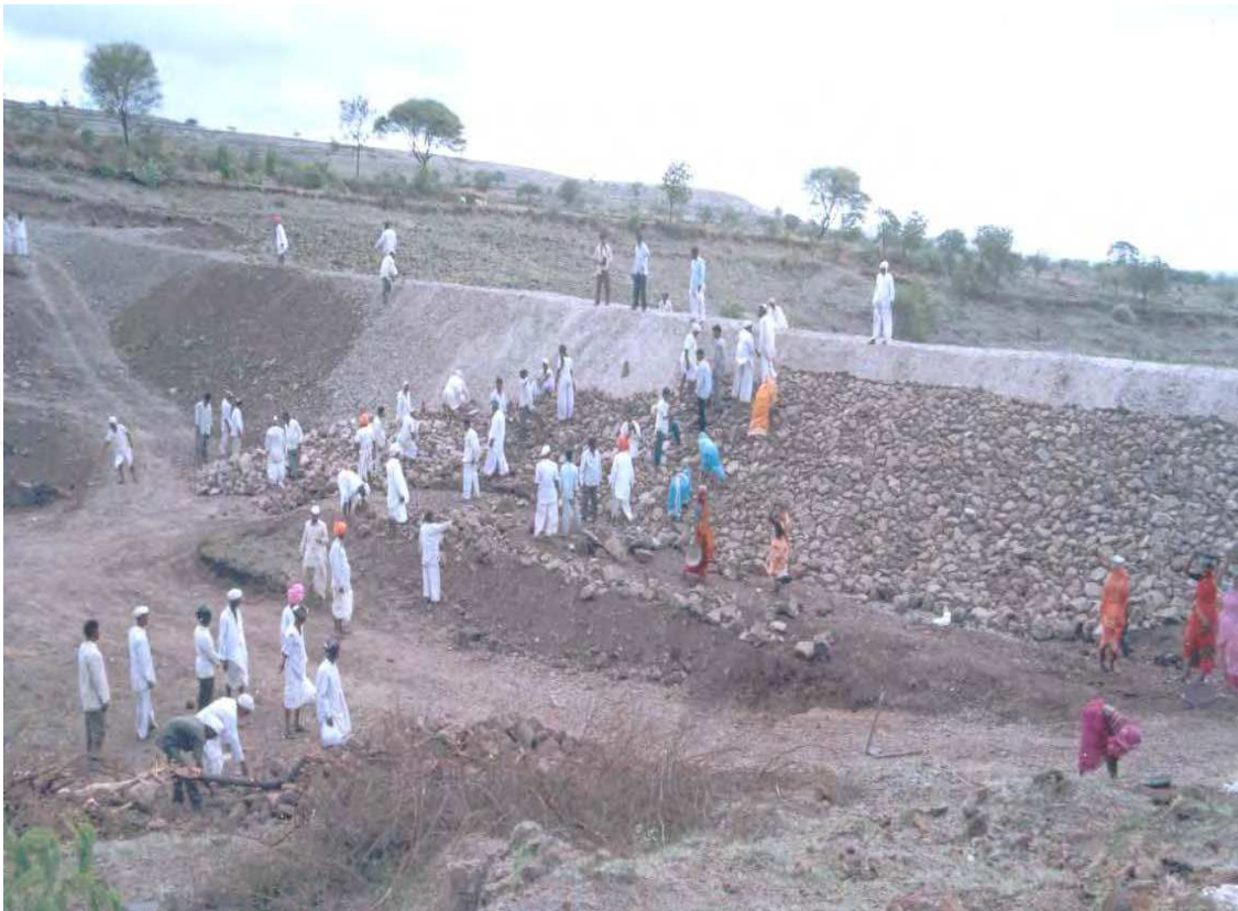
Fig. 5. Stone Pitching on the face of the earthen bund of a percolation tank under construction. Photo from village Hivre Bazar, District: Nagar, Maharashtra state.
