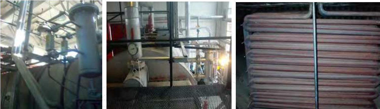
Fig. 3. Superheater of the heat recovery steam generator at 2xST 18 Cogenerative Power Plant
