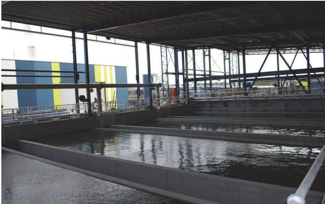
Fig. 25. Gravity dual media filters (Australian desalination plant)
