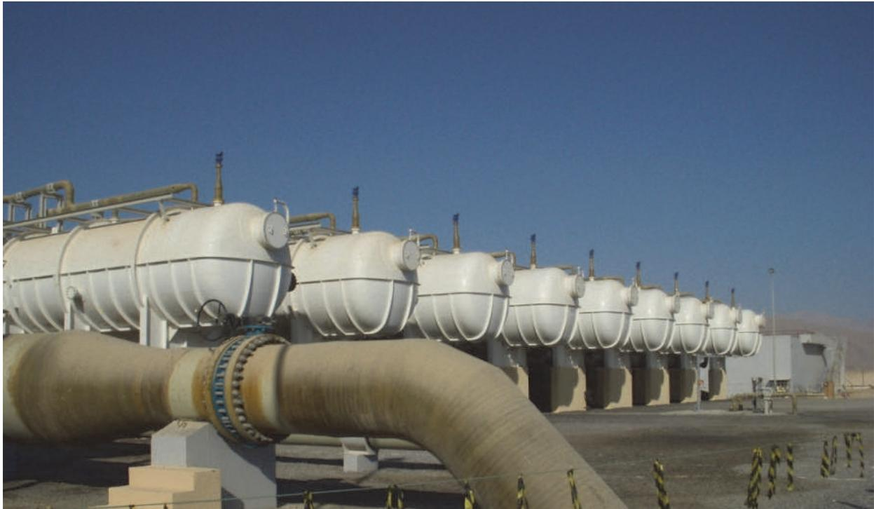
Fig. 24. Single media Pressure filters (Oman Sur desalination Plant)
