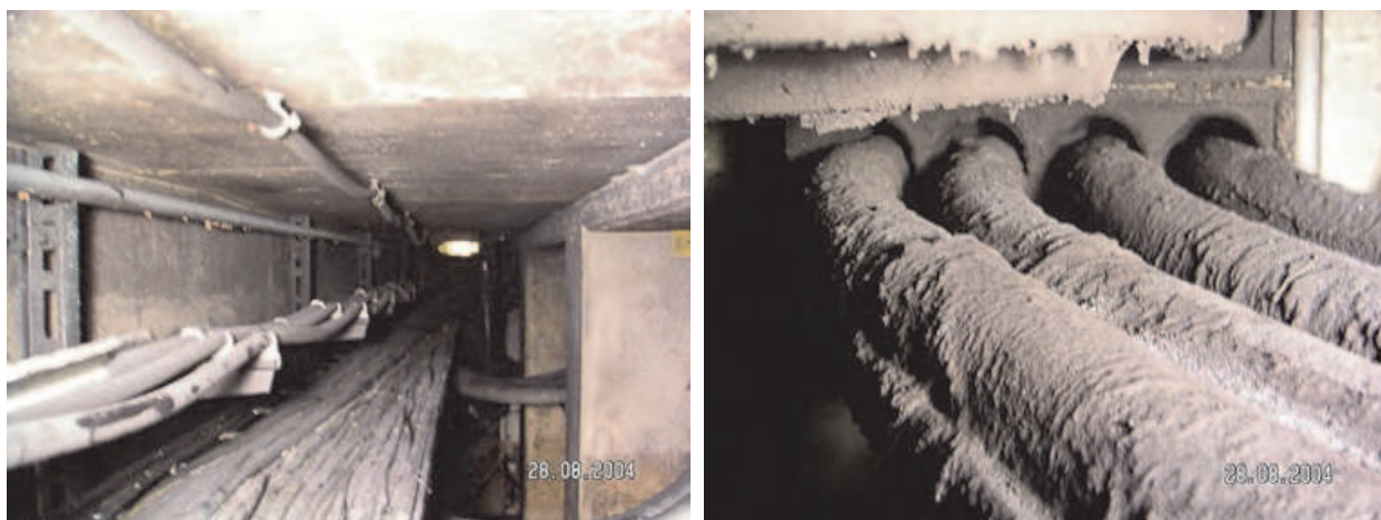
Fig. 4. Cables with protection by intumescent coating; left: photo of the cable channel, right: photo of the coating
