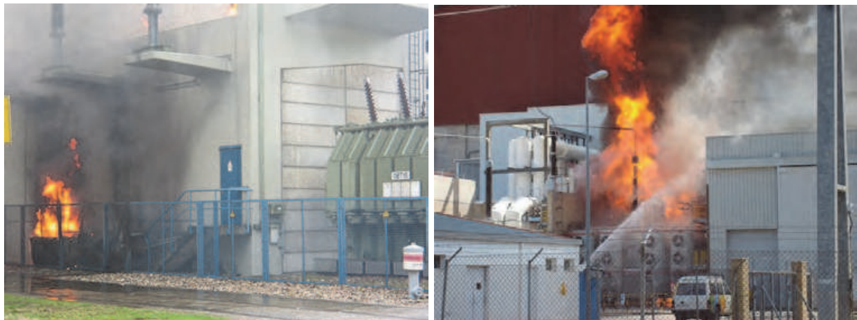
Fig. 8. Flame and smoke occurring at the generator transformer; the photo on the right hand shows the fire extinguishing activities
