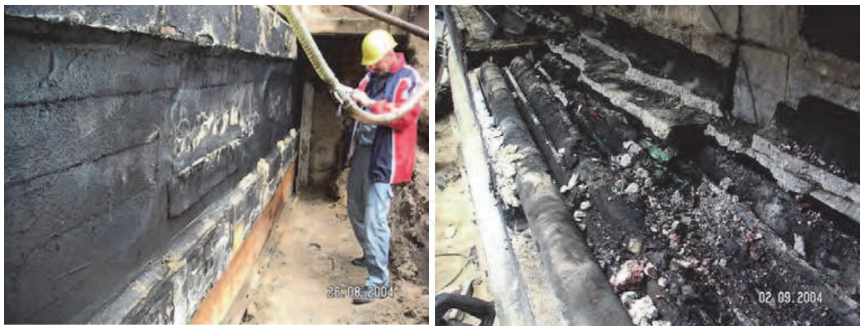
Fig. 3. Photos of the cable damage; left: location of the damaged cable, right: damage by the cable fire/evaporation
