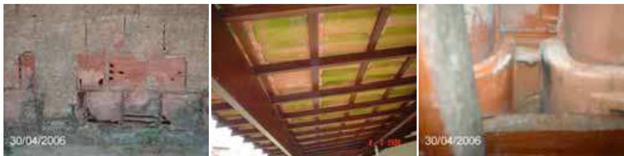
Fig. 1. Fast degradation of masonry and tiles
