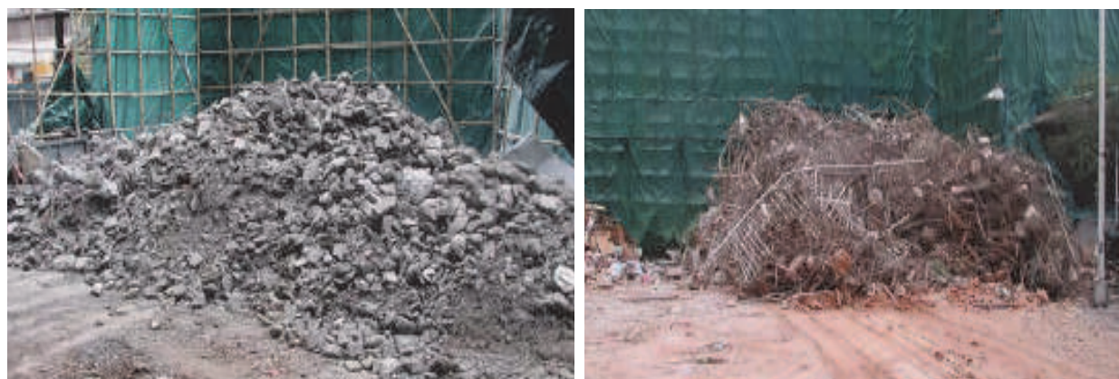
Fig. 9. Sorted broken concrete and steel stockpiled separately (Public Fill Committee, 2004)
