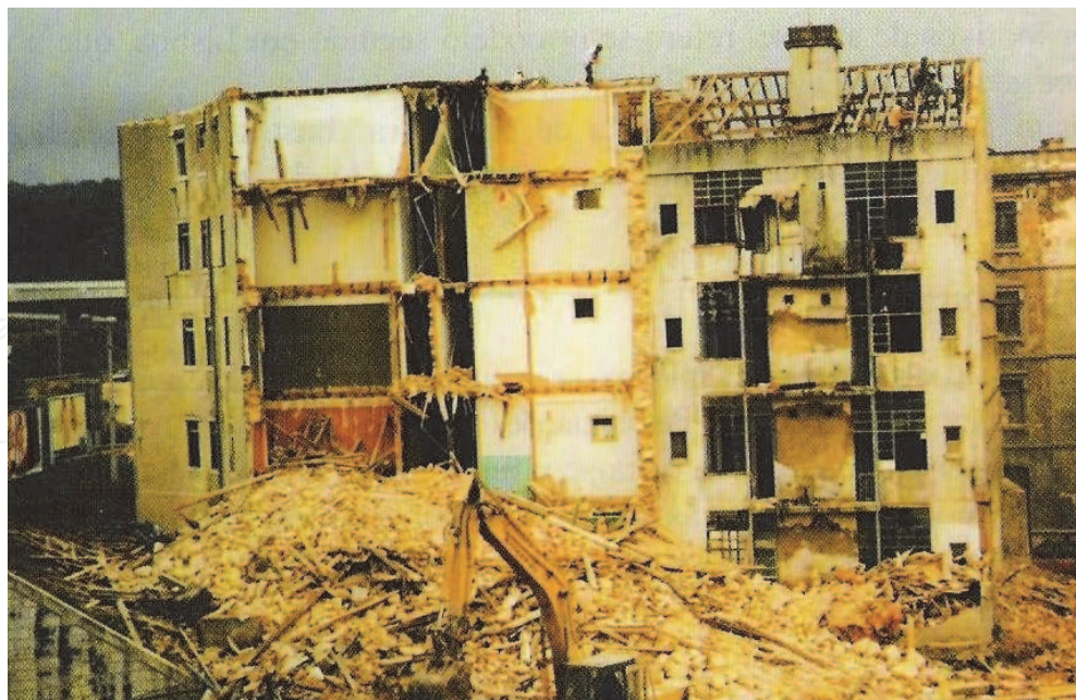
Fig. 8. Sample of an undifferentiated demolition. Source: (Pinto, 2000)
