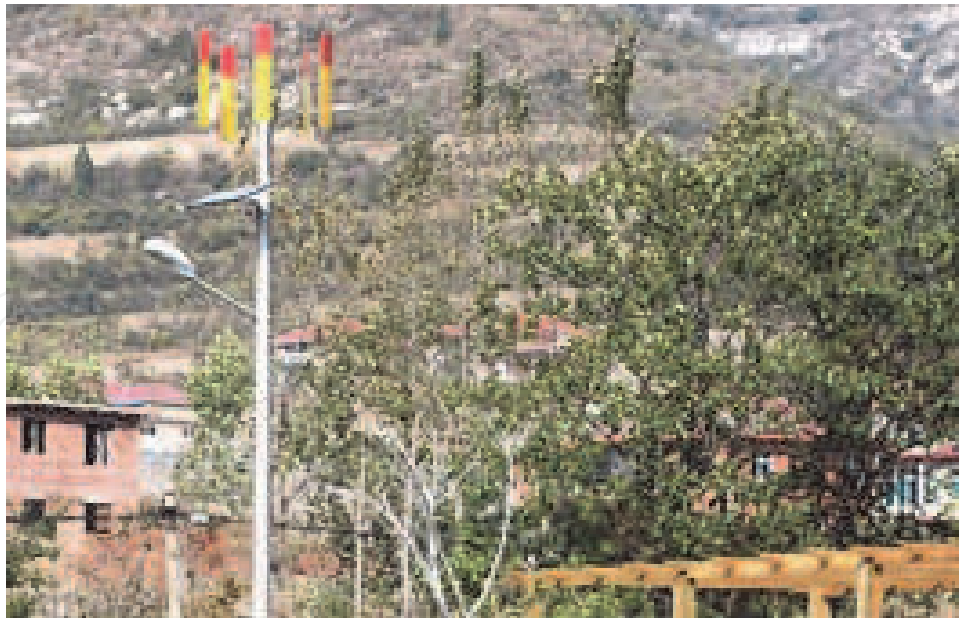
Fig. 7. Magnetically suspended and self-pitched VAWT from Maglev Engineering Center, Shandong University
