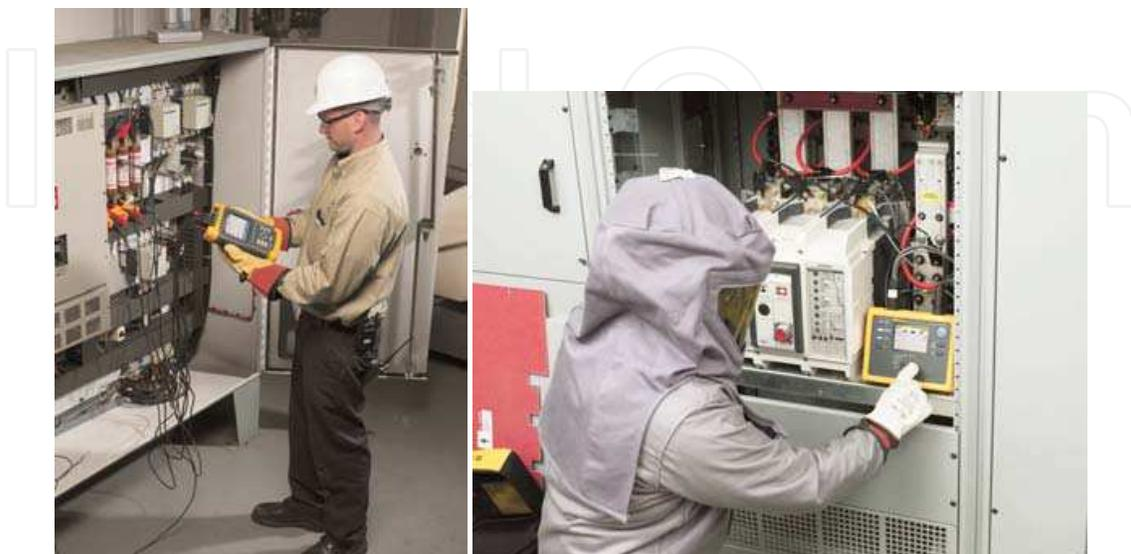
Fig. 5. Measuring in an installation requires several safety measures (Source: Fluke).
