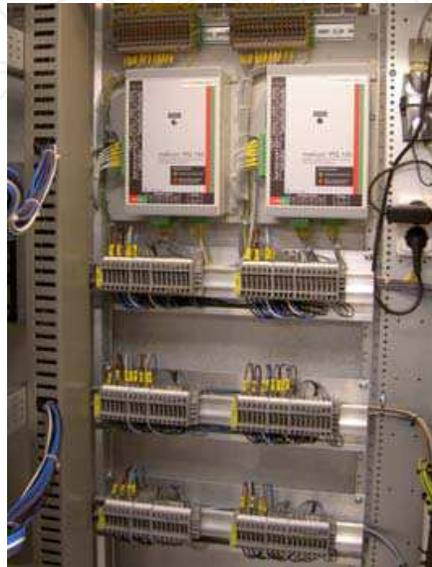
Fig. 8. PQ measurement devices installed in a substation (Source: Metrum)
