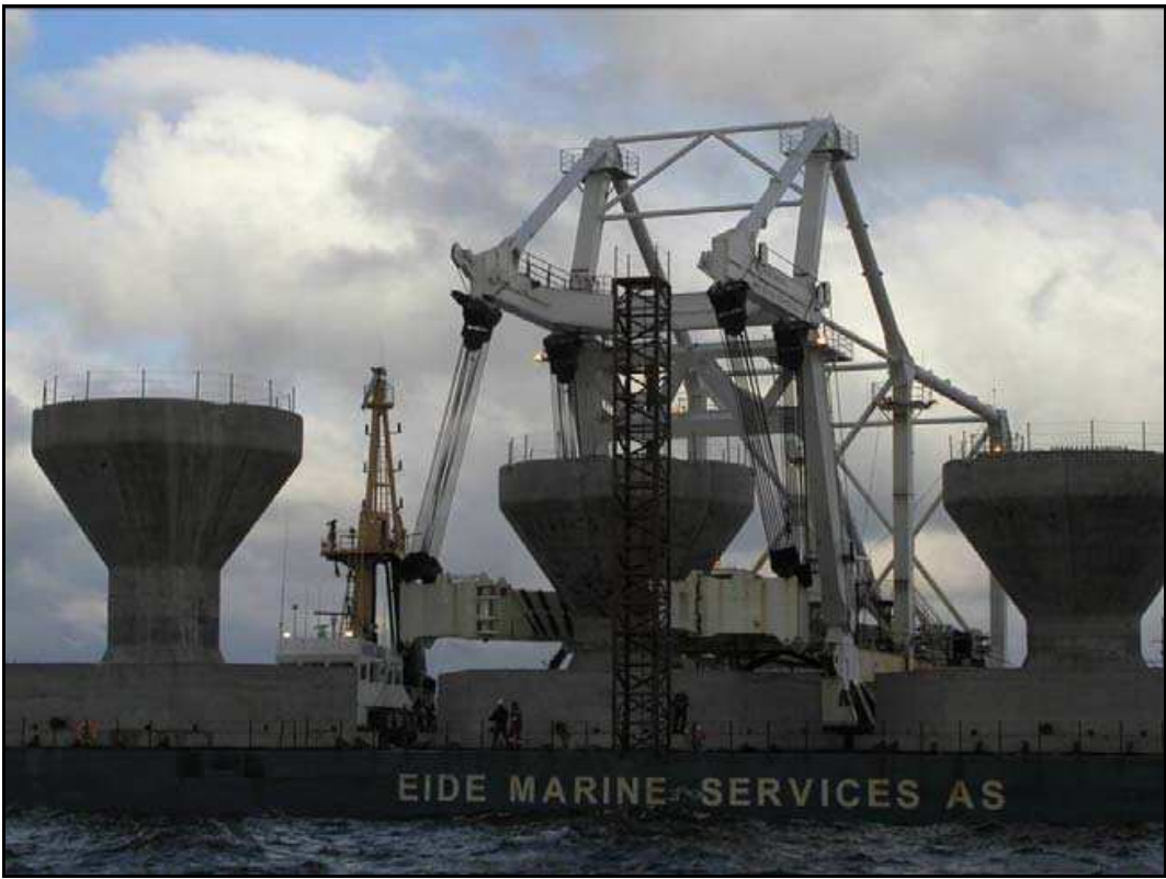
(b) Gravity Bases being lowered from barge
