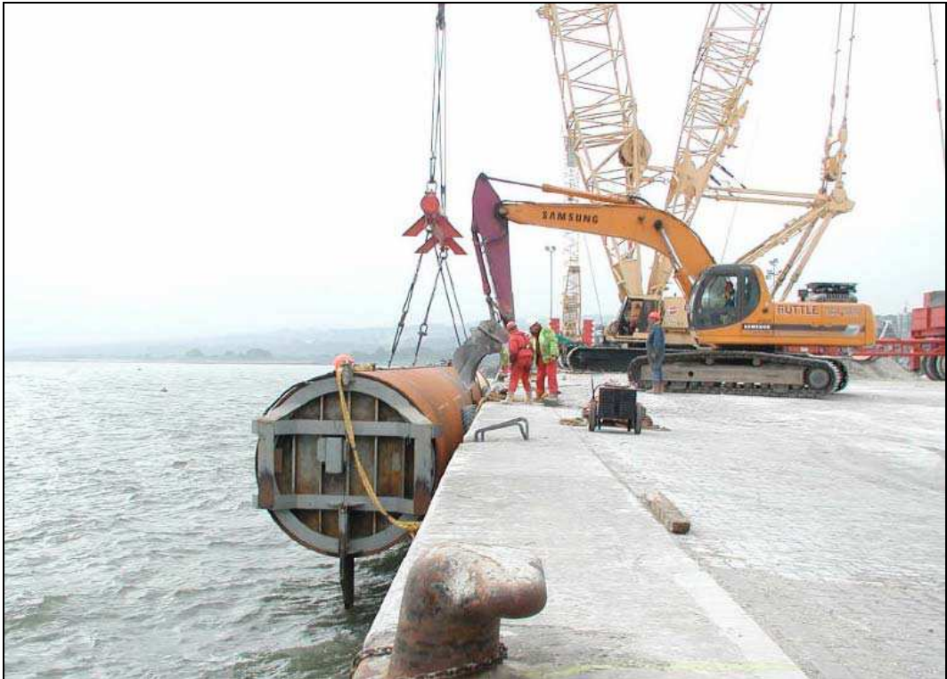
(a) Monopile being floated out to site.
