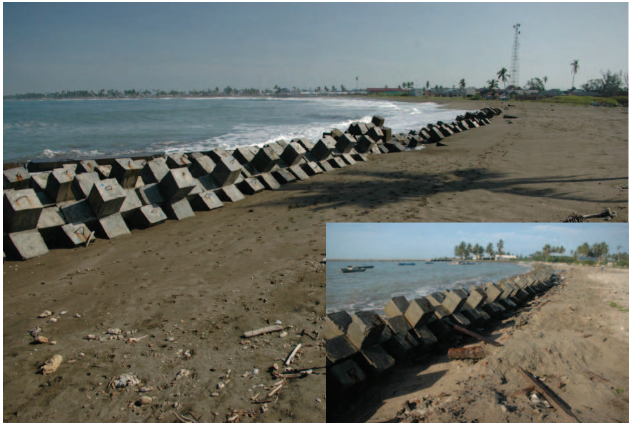
Fig. 8. Protective concrete structures set in place along (a) northern and (b) southern coasts of the Peninsula of Meulaboh. Note that only the southern coasts were actually eroding; along the northern coasts the beaches were accreting.
