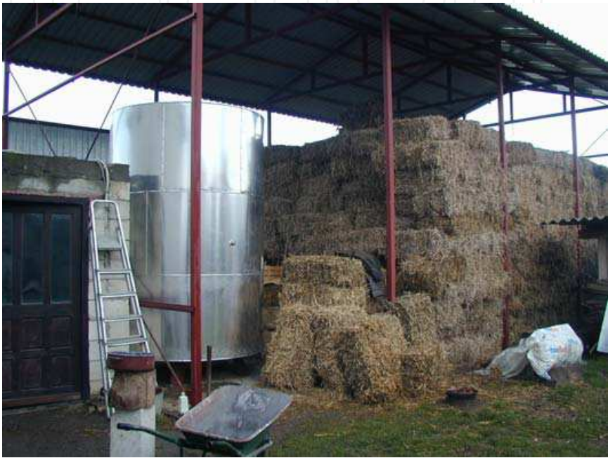
Fig. 6. Heat accumulator (thermal reservoir)
