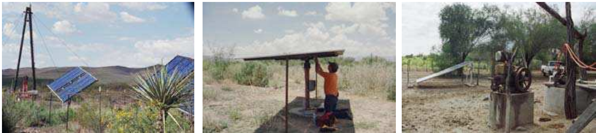
Fig. 4. PV water pumping systems in Chihuahua and Baja California Sur, and FIRCO engineer conducting performance evaluation.
