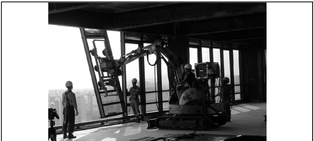
Fig. 2. An ASCI (Automation System for Curtain-wall Installation)
